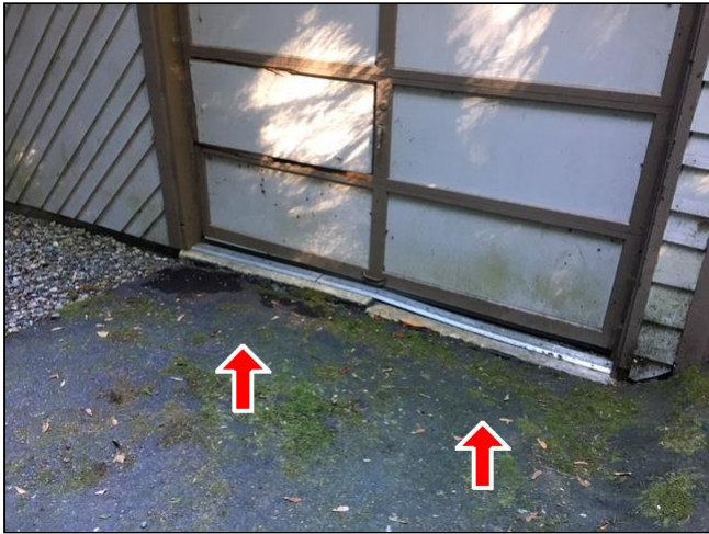
7.0 (1) Garage Door Damage
