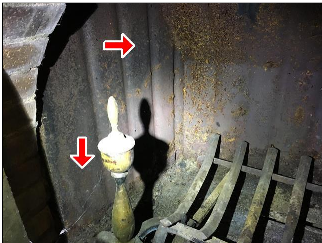
10.5 (1) Firebox corrosion
