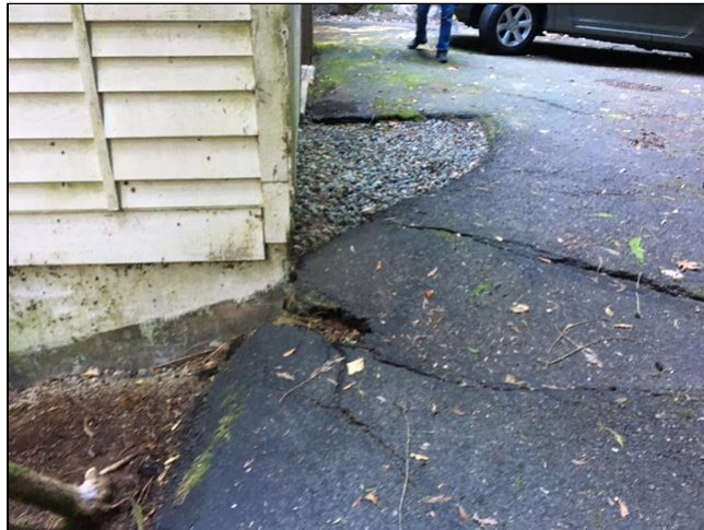
3.1 (1) Deteriorating Asphalt Driveway
