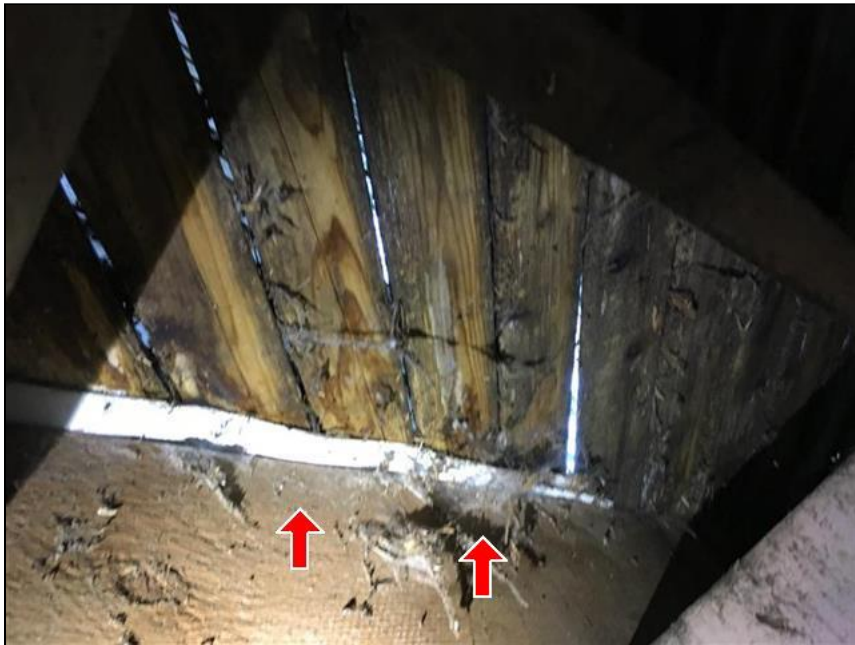
3.6 (3) Rotten Decking from Below
