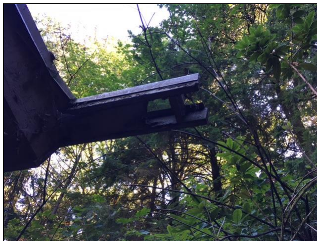
1.3 (1) Failed Cedar Gutters
