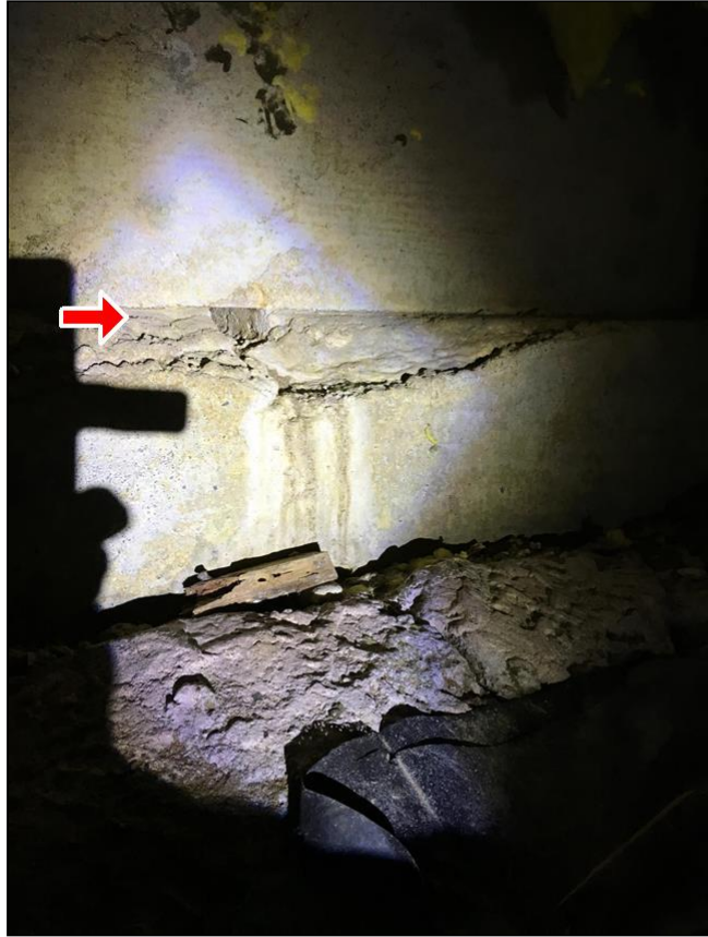
5.3 (1) Concrete Form Holes
