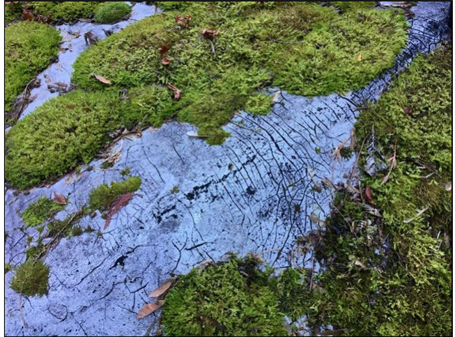
1.7 (2) Heavy Roof Cracking
