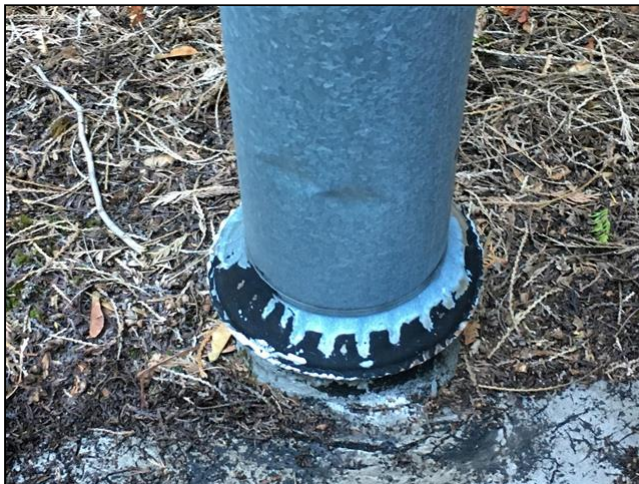
1.2 (1) Repaired Flashing
