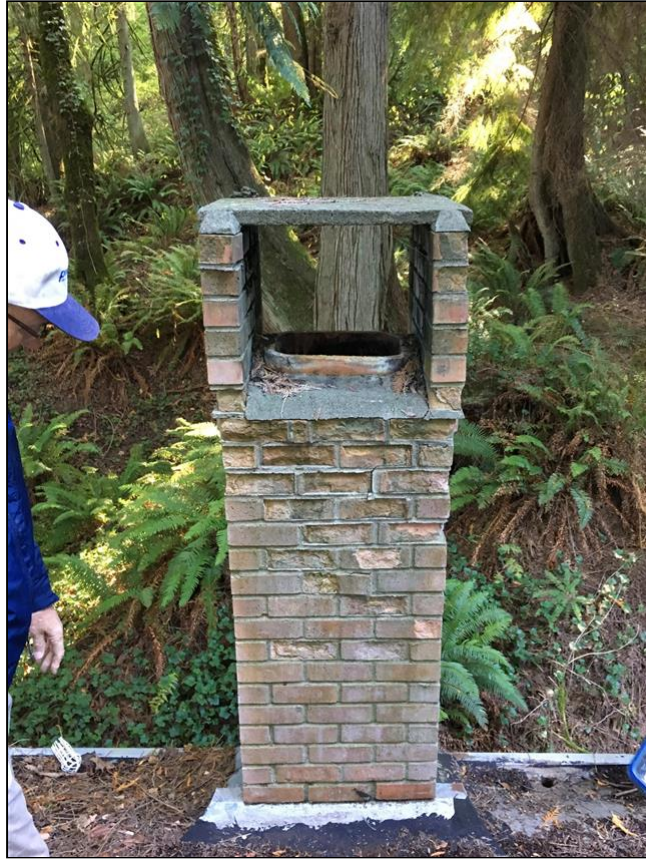
1.5 (1) Chimney at the roofline
