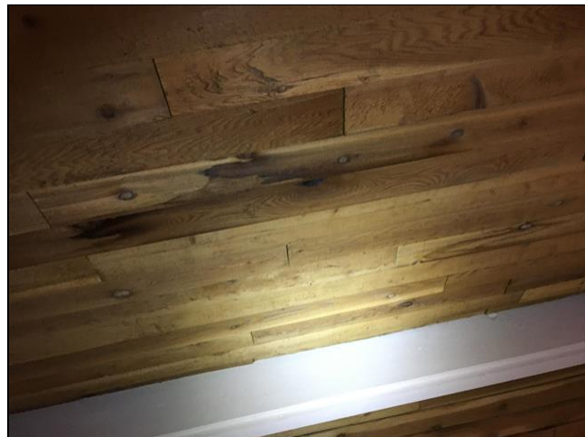
8.2 (1) Roof Leak
