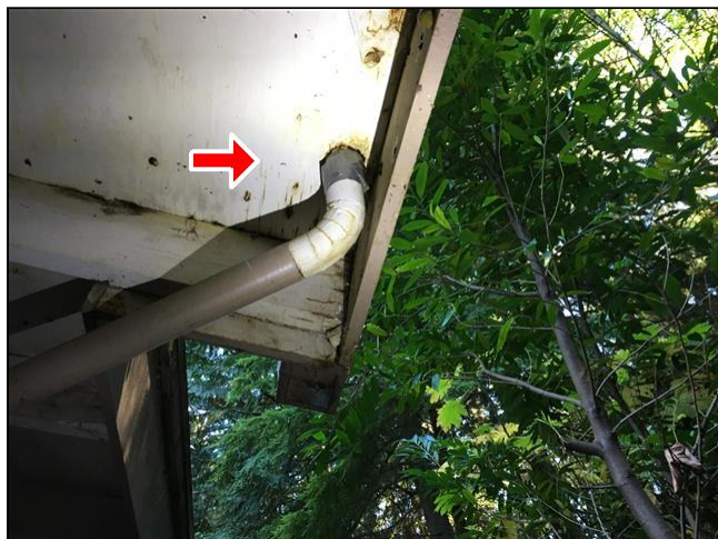
1.3 (2) Failing Gutters
