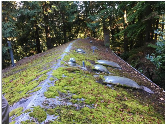
1.0 (1) Heavy Moss on Roof
