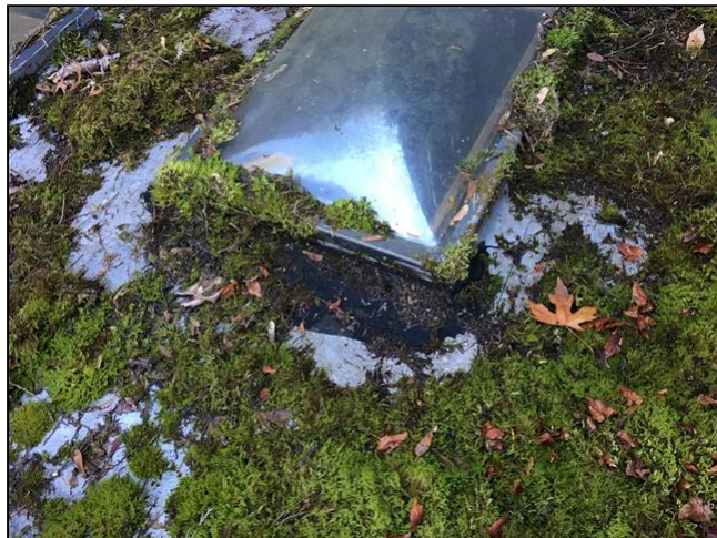
1.6 (1) Skylights - no flashing
