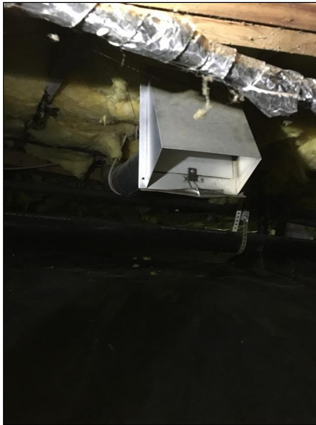
12.13 (1) Venting to Crawlspace
