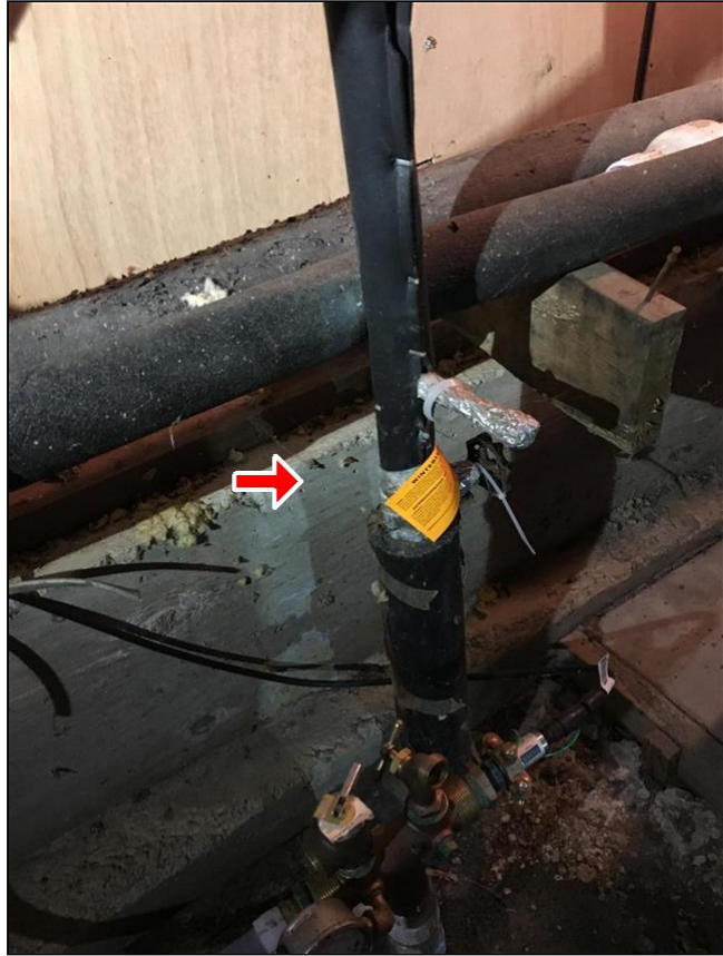
9.1 (1) Main Water Cutoff in Crawl Space
