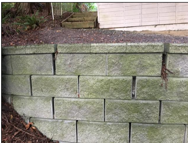
3.7 (1) Retaining Wall Settlement
